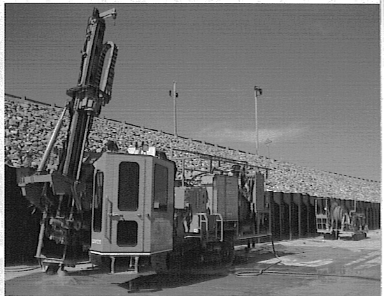
Figure 2. Contemporary drilling rig installing inclined holes.
